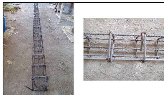
Fig. 5. Reinforcement cage for conventional beam
