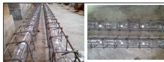
Fig. 6. Reinforcement cage for voided beam without spacing
